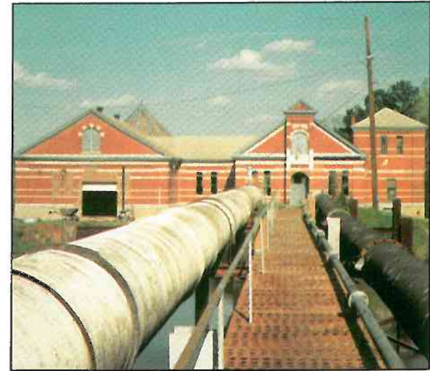
Above: The Augusta Water Works, at mid-canal, is an outstanding example of 19th century municipal architecture whose function has been continuously linked to the Canal. (JV)
