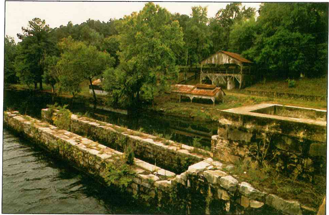
Above: At the Headgates area, the 1845 lock and Canal can be seen against the backdrop of the hill which marks the Fall Line. In the background are the WPA-era dance pavilion and barbecue pit. (AC)
